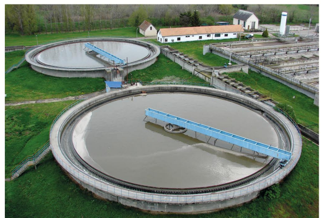
[5] Dorr-type settlers (foreground) and biological wastewater treatment basins (in the background)
