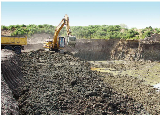
11 Remediation of a former military airfield: cleaning of oil polluted soil and groundwater
