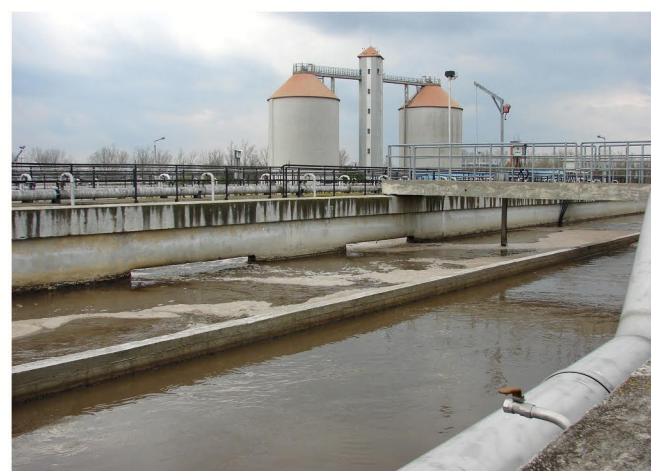
[6] Biological sewage treatment with activated sludge system, with putrefactive towers in the background
